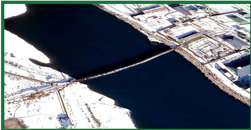
(Figure 6.10.5: Satellite imagery of the footbridge connecting Shiveh in Afghanistan to Khorog in Tajikistan. Marked as Location "4" in Figure 6.10.4)
