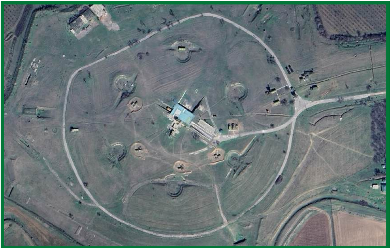
(Figure 6.5.8: Satellite photography of Tajik air defence batteries just west of Dushanbe)
